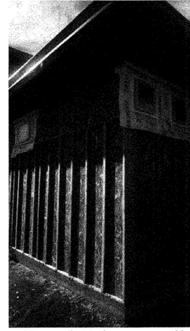
In this example 2 inch spacers are added to the exterior air barrier. Insulation is only required on the interior side of the air barrier not between the spacers.
