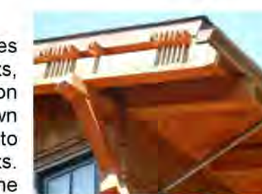
Building with copper flashing, gutter and drainpipe.
