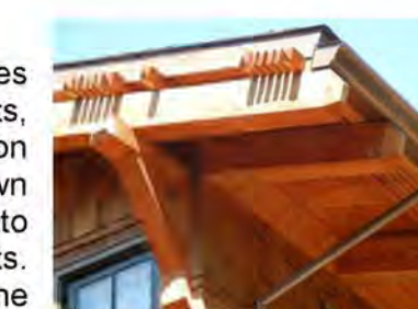
Building with copper flashing, gutter and drainpipe.
