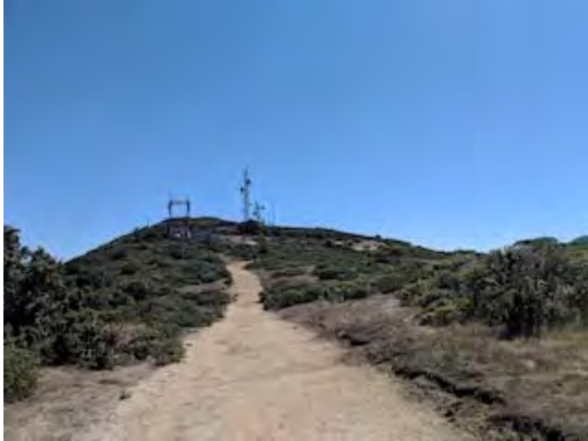
View of existing access road and cellular facility.
