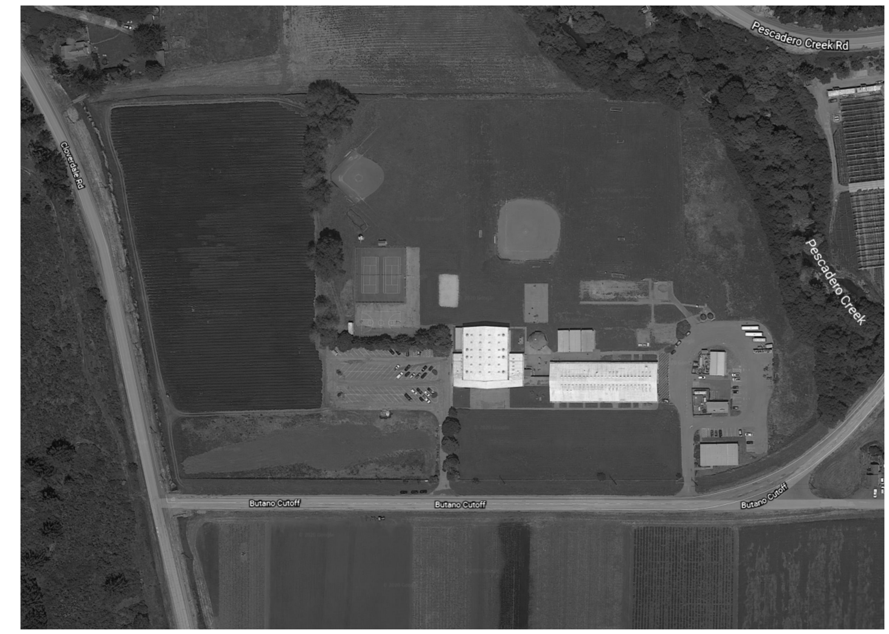
Existing La Honda High School Site
