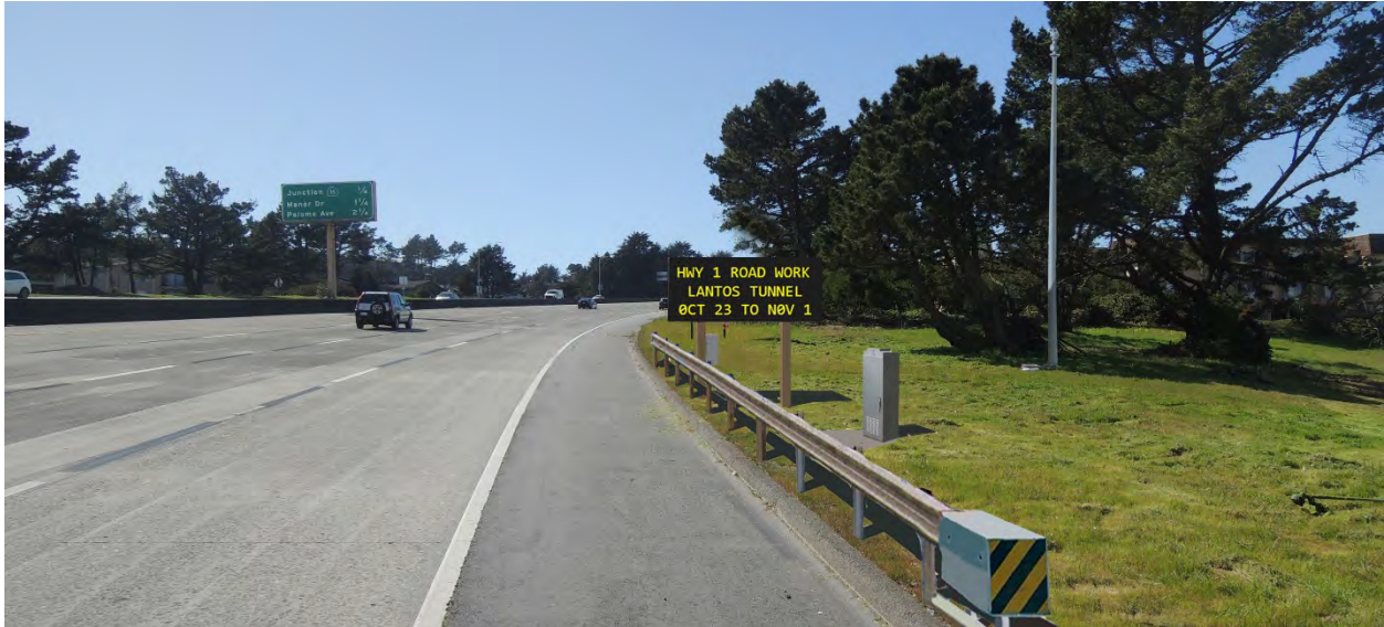
Figure 1-32 Visual Simulation of VMS (shown with message displayed) and MGS at Location 10
