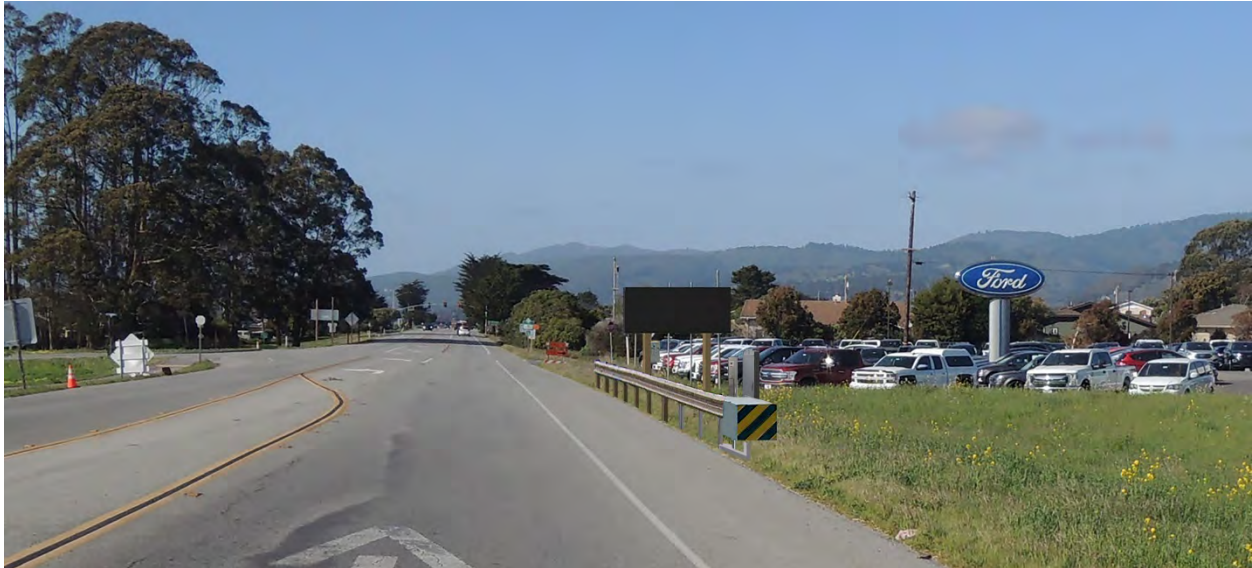
Figure 1-6 Visual Simulation of VMS (shown without message displayed) and MGS at Location 2
